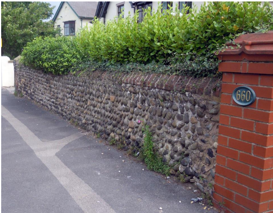
Historic cobble wall
