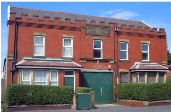
Former drill hall, Talbot Road
